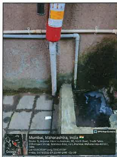
Waste Water In Seepage Tank
